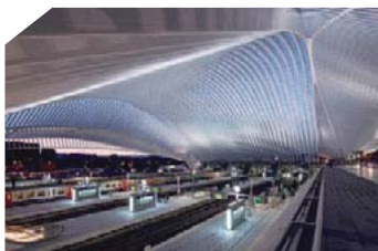
High-speed train station Liège - Belgium
