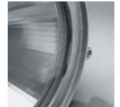
Slots allowing rainwater to run off
