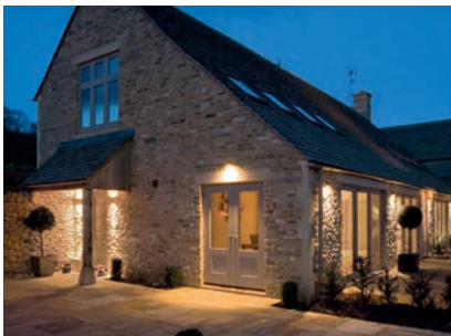
Location: "Hills Farm" - London sub. (UK) Project: Lightmaster Direct Ltd
