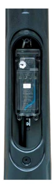
Connection box installed in plastic coated pole
